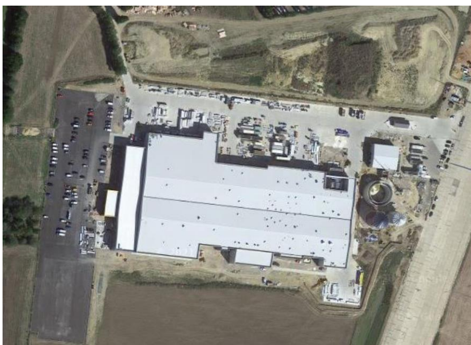
Figure 1. View of Cranswick PLC Eye site.
